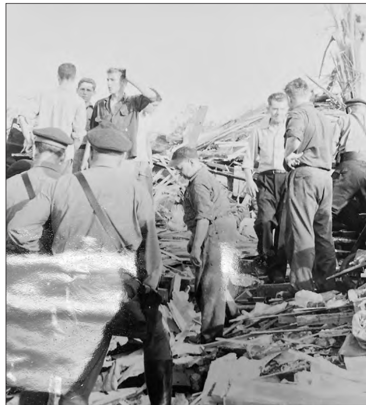
The 1953 Tornado destroyed this two tenement house on Old Stage Coach Road in Barre.
