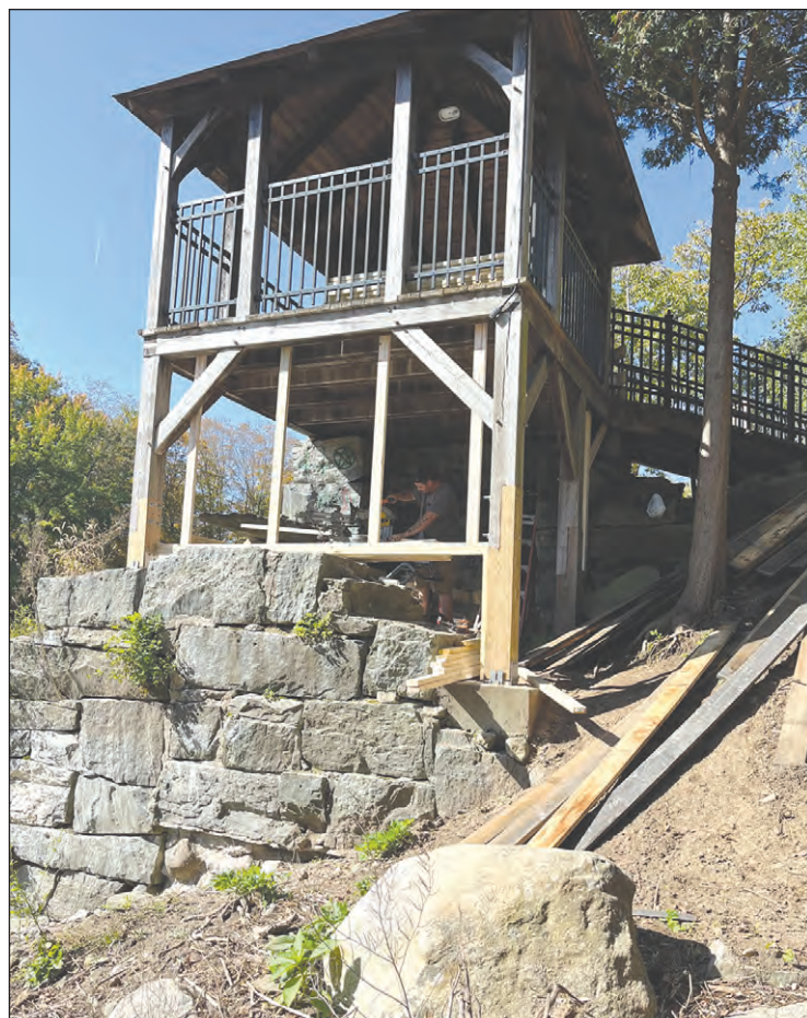
Repairs were made to replace rotting posts on the gazebo.
