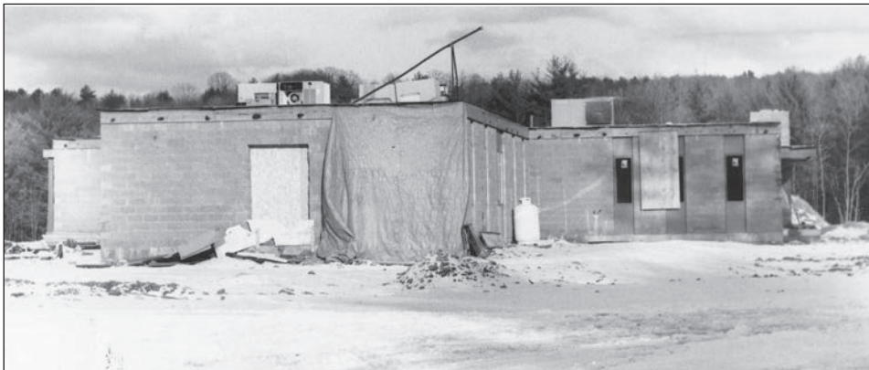
Much progress can be seen on the construction of the Barre Health Center, Worcester Road, Barre on Feb. 29, 1984.
