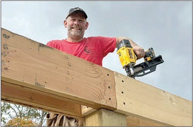
Matt Koziol attached the blocking brackets between the beams.
