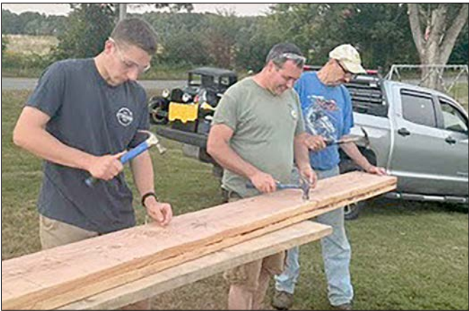
Ethan Salvadore, Dennis Letendre and John Head nailed boards together to create the beam to span the front opening of the pavilion.
