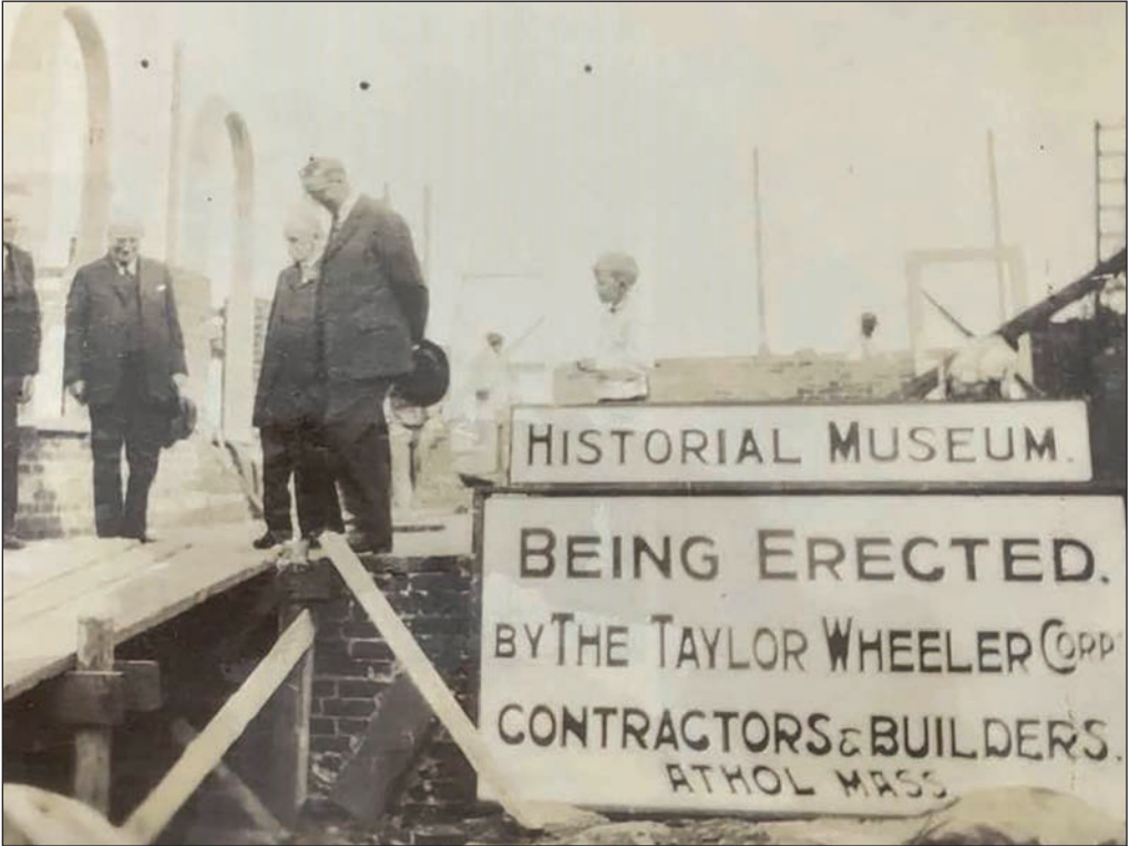
This photo is of construction on the Petersham Historical Society Building.
