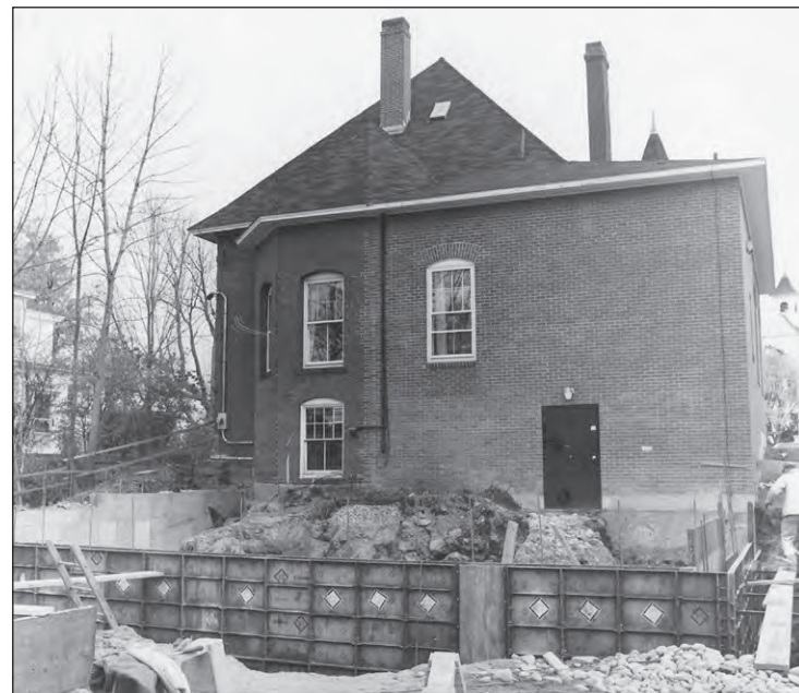
On Oct. 30., 1985 the Barre Savings addition begins construction.
