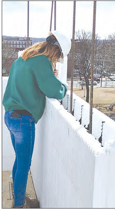
Submitted photo Dean student working with rebar at Chestnut.
