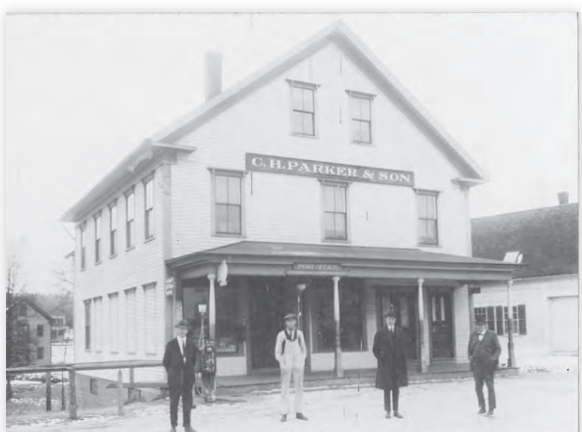
C.H. Parker and Son General Store was located in the Coldbrook section of Oakham. Parker also owned a sawmill.
