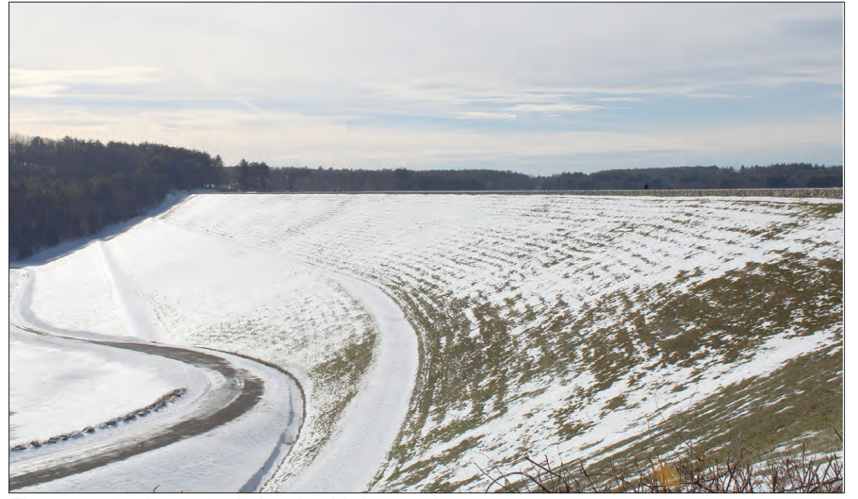
There are 40 caissons buried under this impoundment.
