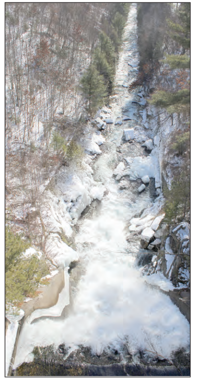
The lower spillway creates a waterfall, and only releases water when the Quabbin Reservoir is at or near capacity.
